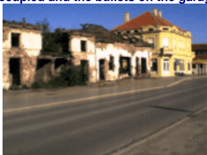
Notice the yellow building has been refurbished, as it was worse than the others!
